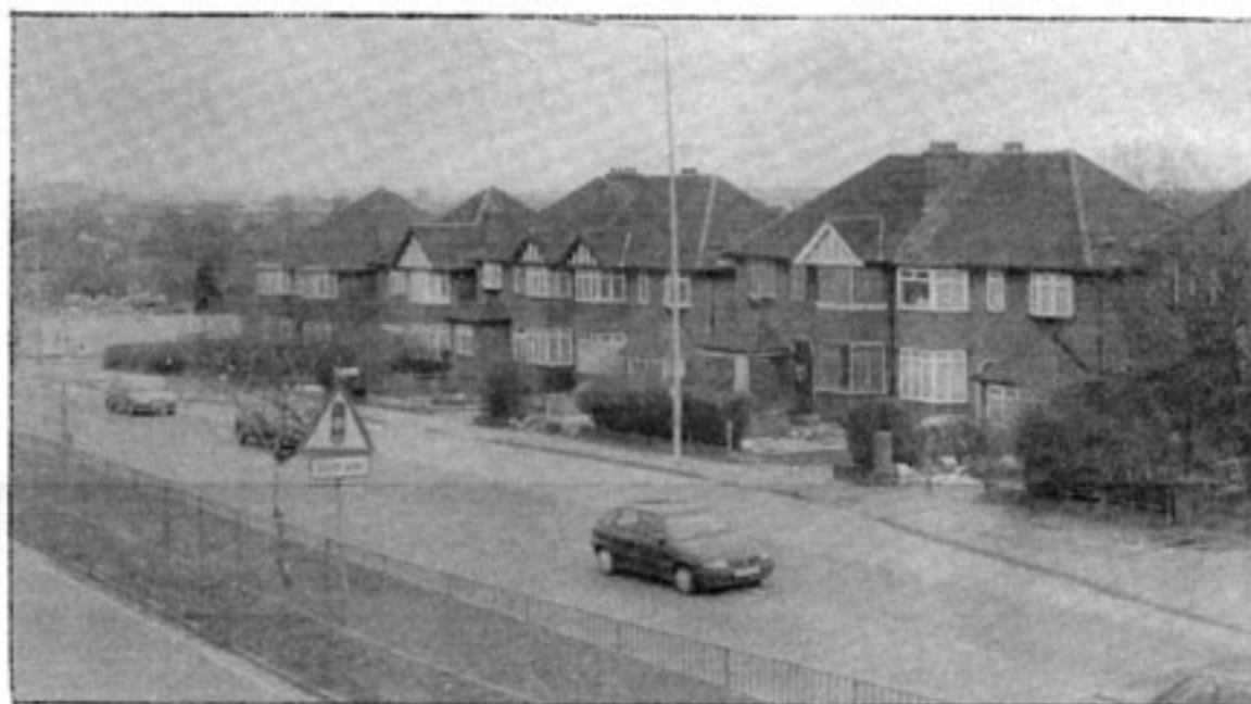
Homes on Western Avenue boarded up before they were demolished.
